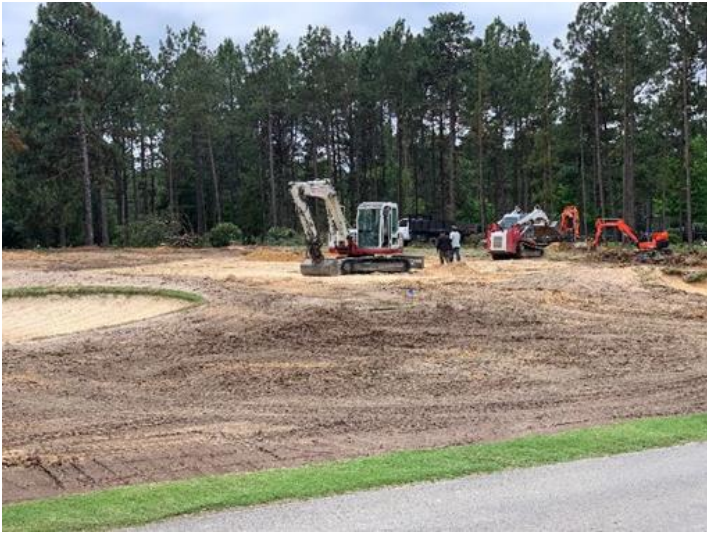
The short game area has been stripped of all grass. The new green and bunkers will be repositioned and shaped in the coming days.
